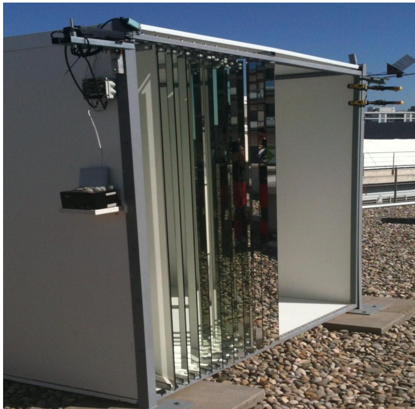
Figure 34. The reflectors facade: During the installation of the concentrating PV façade at the Applied Energy Research Centre (CREA) at the University of Lleida (Spain). The tracking system is noticed on the left.
