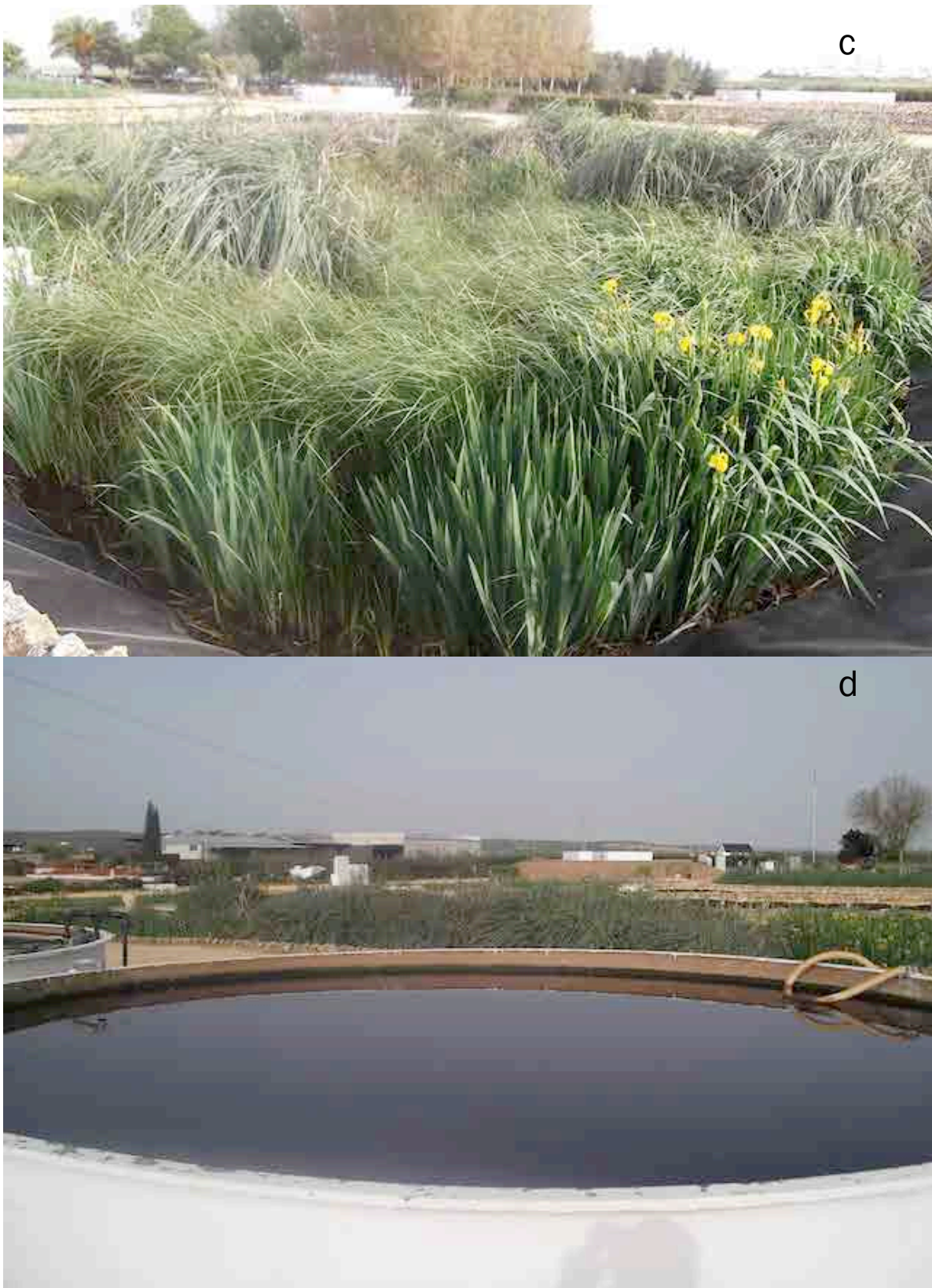
Figure 7.2. View of the different units of the pilot hybrid treatment system: vertical subsurface flow (a); horizontal subsurface flow (b); free water surface wetland (c); water tank for reuse (d).
