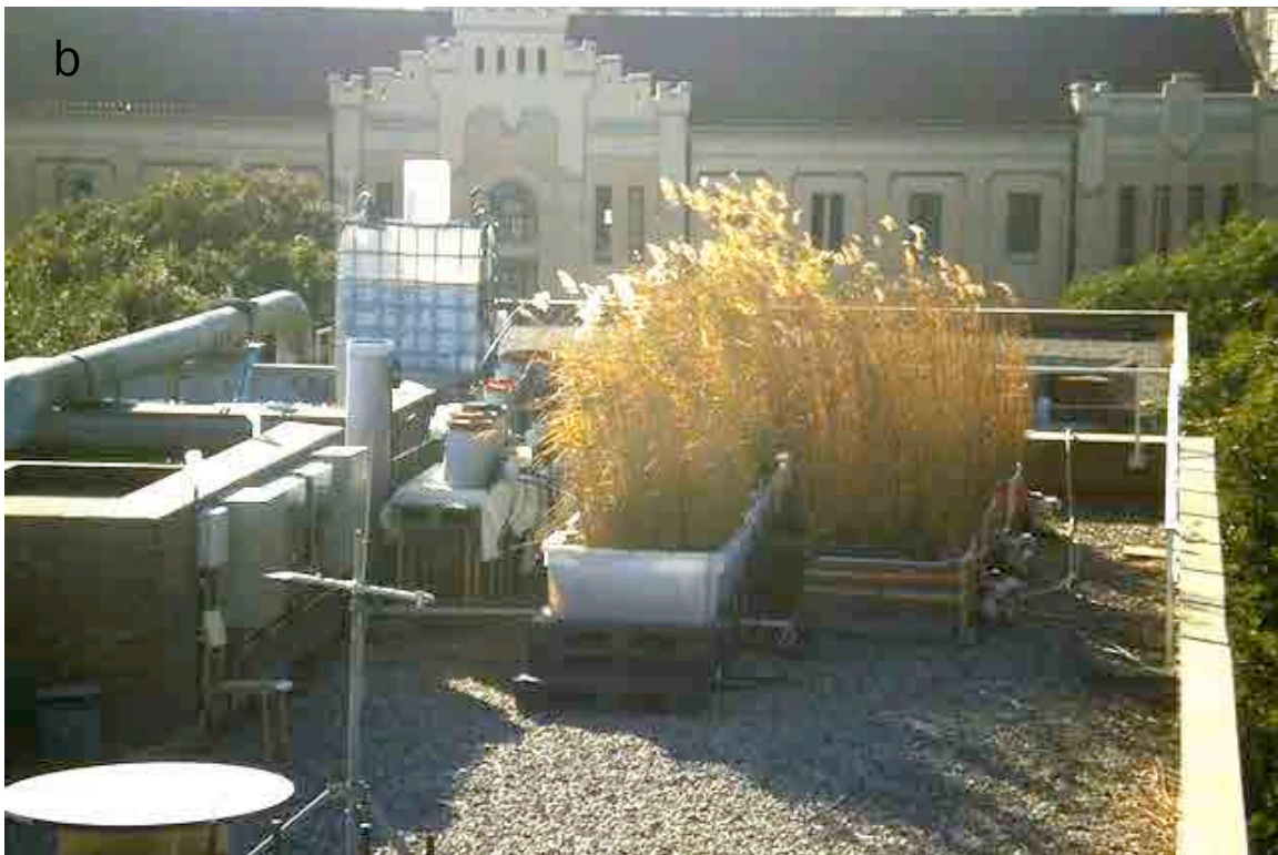
Figure 4.2. View of the experimental horizontal subsurface flow constructed wetland system in Barcelona. a) summer; b) winter.
