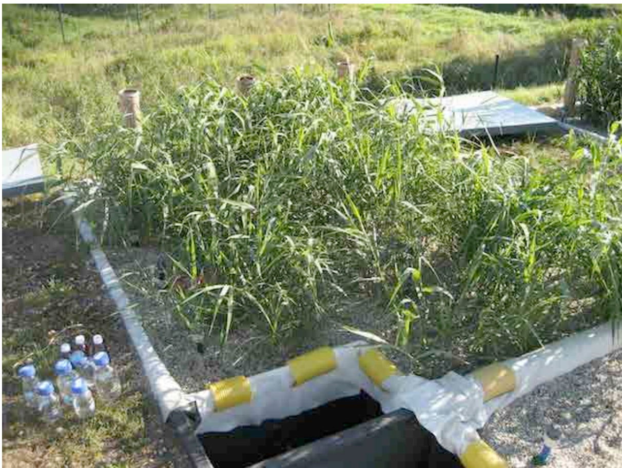
Figure 9.1. View of one of the pilot-scale vertical subsurface flow constructed wetlands of the experimental wastewater treatment facility of Langenreichenbach, Germany.
