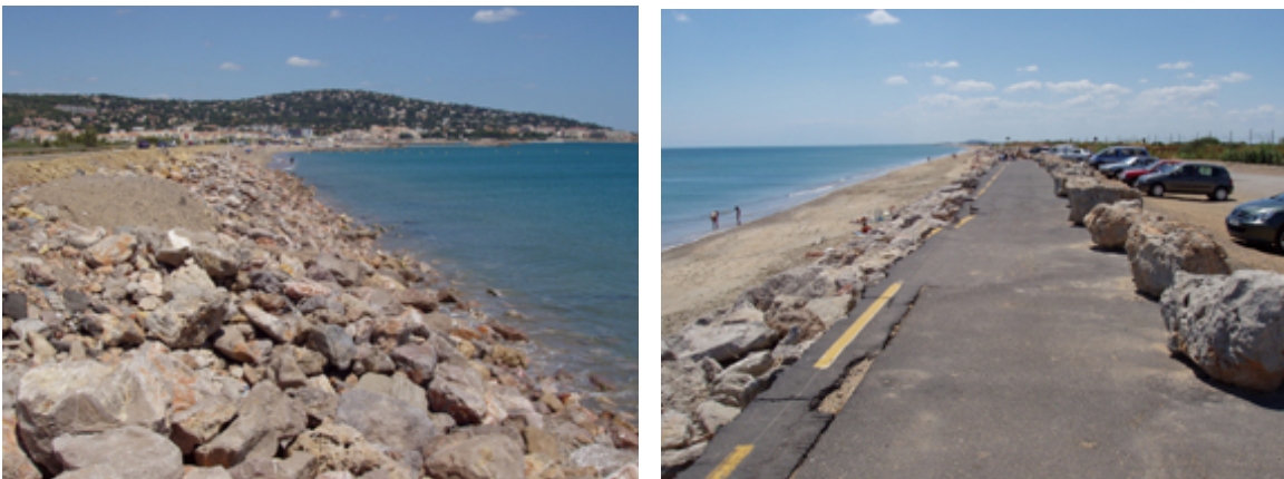
Figure 8.9. Wall protection for road.
