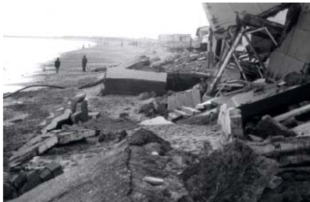
Figure 8.10 Illustration of the effects caused by a coastal storm in 1982. Source: Urbanis (2004).
