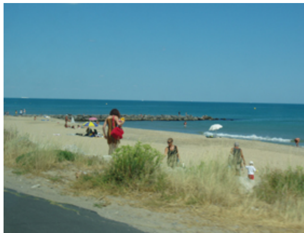
Figure 8.7 Groin northwards of the camping Le Castellás.
