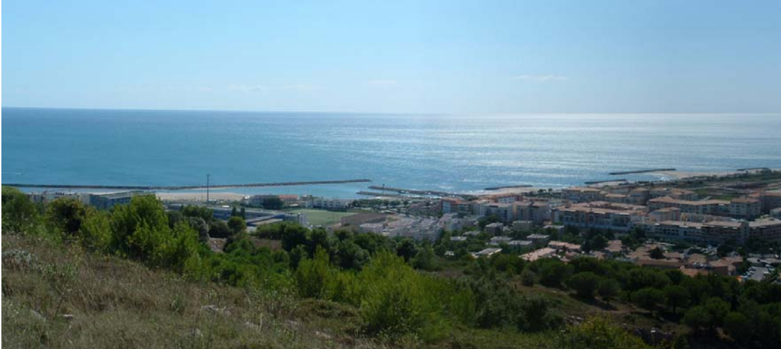
Figure 8.8 View of the coastal defences in the Lazaret beach and the marina of “Quille’s” mouth. However, the effectiveness of these coastal protection measures has been questioned because of their negative impacts downdrift of the last breakwater, showing a high erosive trend, especially intensive in the section where the coastal road is close to the beach. (See Figure 8.9)
