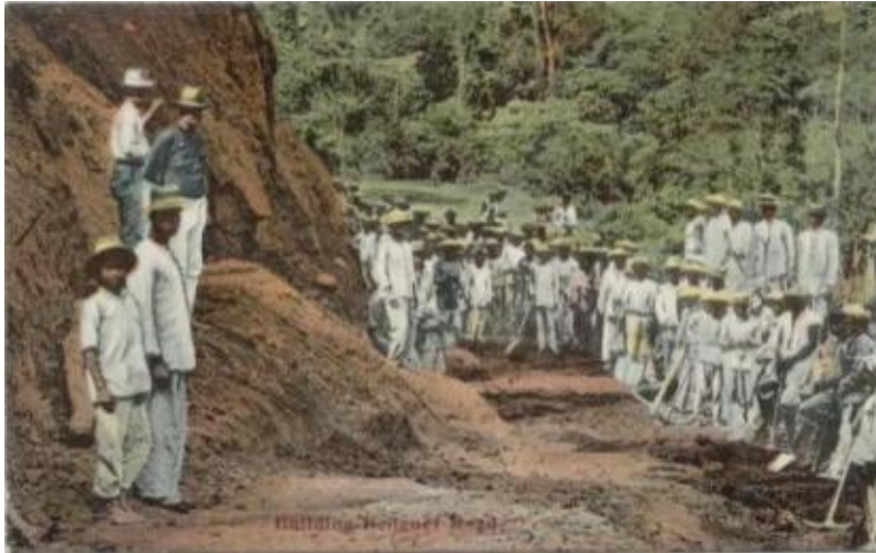
"Building the Benguet Road" Font: E.C.McCullough & Co., Manila, 1901
