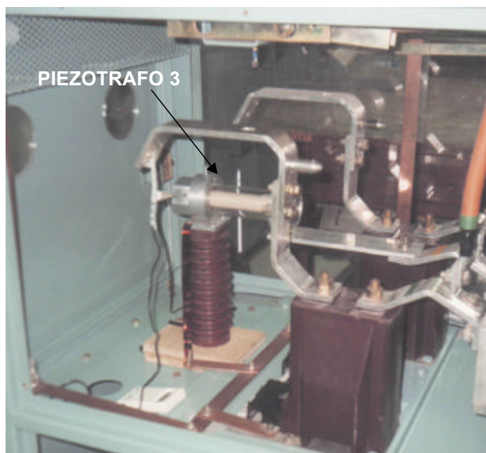
Figure 8.17. Arrangement of the prototype inside the H.V. cell
