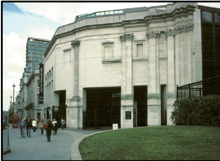
Figura ‘x’. Venturi, Scott Brown & Associates, Sainsbury Wing (1991). Londres.
