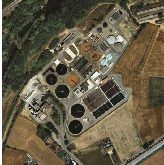
Figure 5. Installations of WWTP TRARGISA at Girona, Catalonia, Spain (source Google maps).
