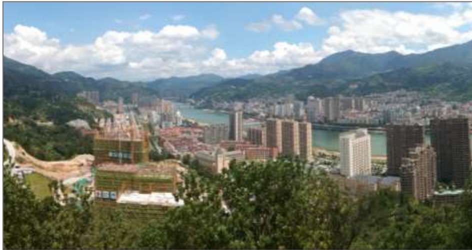
Illustration 3: Nursing home under construction in Shuinan (Qingtian).
