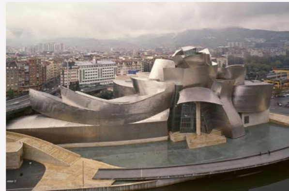
Figure 4. Left and bottom right: Groundplan of first floor and view of the Guggenheim Museum in Bilbao by Gehry Partners, 1991-1997. (left) Image Source: "Les Infos Du Paradis, Kurt W. Forster (bottom right) Image Copyright: David Heald
