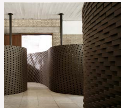
Figure 5. View of Structural Oscillations presented in the 11th Venice Architectural Biennale. Images of the brick wall has been assembled on site by a mobile robotic arm (R-O-B Unit). Image Courtesy: Gramazio and Kohler Research, ETH Zurich
