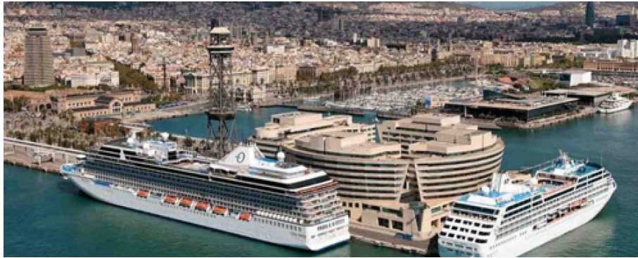
Figure 23. View of North and South terminals. These terminals, according to the agreement of 2018, will be dismantled once the concession finishes. Source: (AQR-Lab Universitat de Barcelona 2016).
