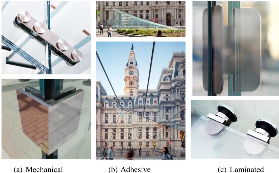
Figure 18. Examples of (a) mechanical, (b) adhesive, and (c) laminated connection in laminated glass elements [1].
