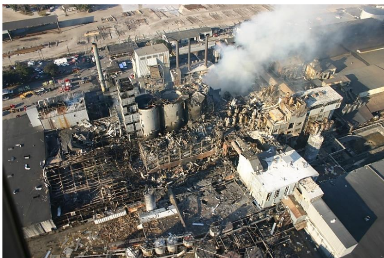
Figure 25. Consequences of a dust explosion in a sugar refinery. 26
