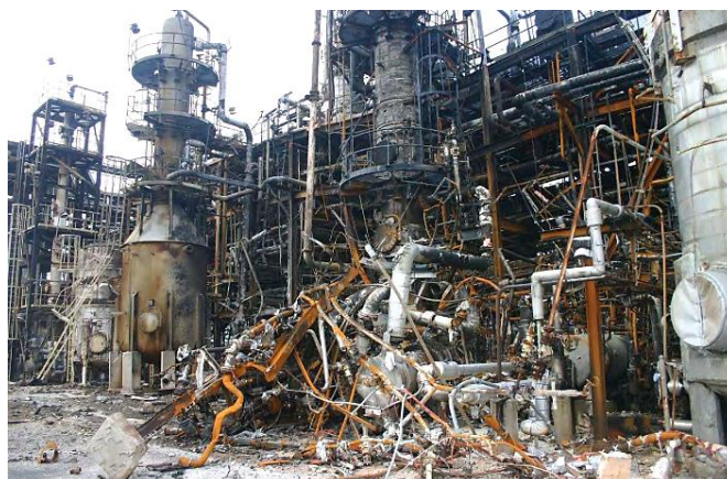
Figure 28. Effect of a runaway explosion in a pesticide plant. 31
