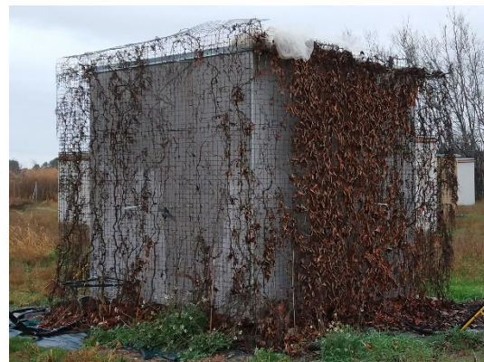
(e) Green facade in winter
