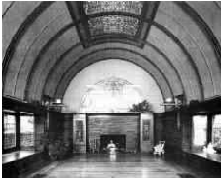
Wright House, Playroom addition, 1895 -98. Interior, looking east, (Levine, 1996, p. 24.)
