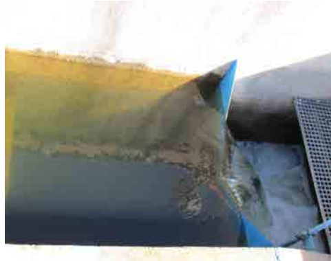
FIGURE 2.18: V-notch weir
