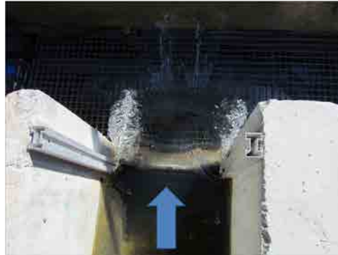
FIGURE 2.20: Top view of Weir 4
