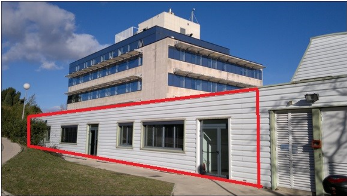
Figure A-1: Renovated building at SupAgro.
