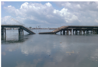
(a) Broken bridge
