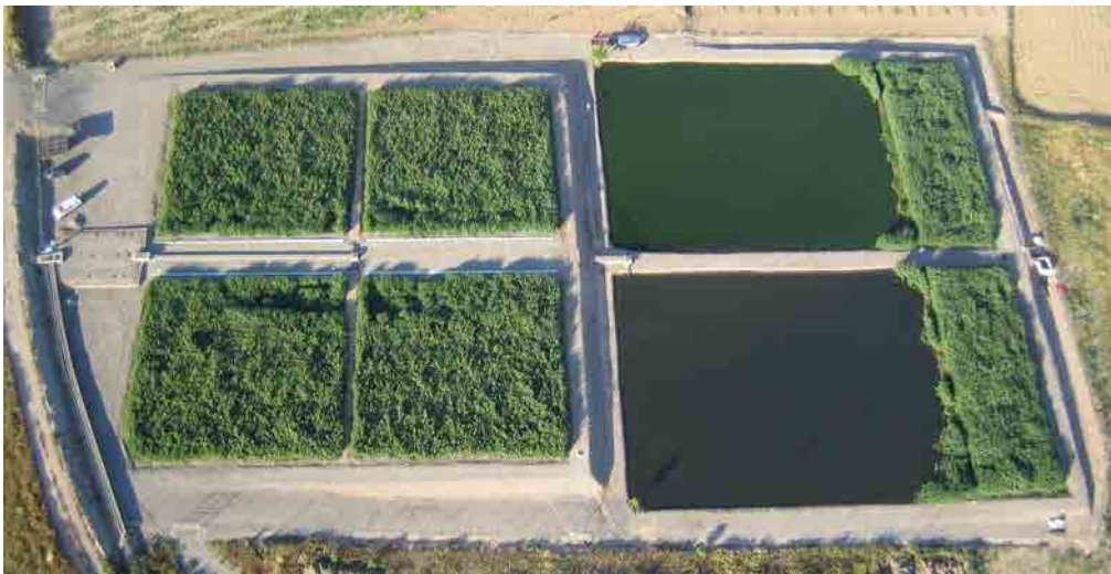
Figure 1.2: Treatment plant based on Constructed Wetlands technology (Verdú, Catalonia). The treatment line consisted on three septic tanks in parallel followed by four parallel horizontal subsurface flow Constructed Wetlands and two surface flow wetlands.
