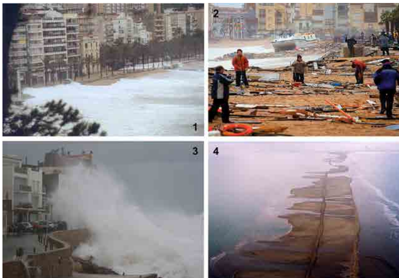
Figure 4.13: Examples of damages caused by storm-induced inundation in the Catalan coast (Location, date and image property). 1: Lloret de Mar (La Selva), November 2001, Lloret de Mar Council; 2: Blanes, December 2008, La Vanguardia newspaper; 3: L'Escola (Alt Empordà), December 2008, Lloret de Mar Council; 4: Ebre delta (Montsià), November 2001, D.G. Costas Tarragona.
