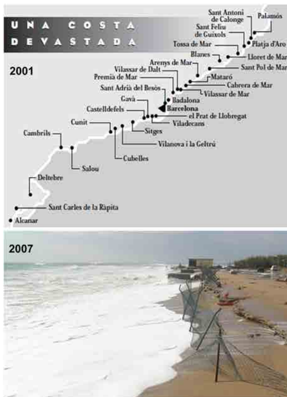
Figure 1.1: Top: Locations reporting damages along the Catalan coast produced by a storm on 2001 (Avui, November 13th 2001); Bottom: Facilities of a desalination plant damaged by a storm on 2007. Blanes, central coast (LIM, UPC).
