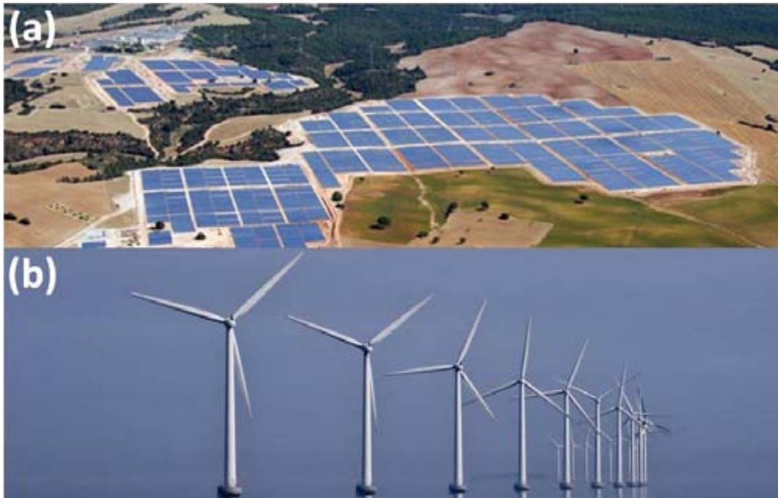
Fig.1. 1. Examples of large scale energy harvesting installations: (a) aerial view of the photovoltaic park in Olmedillas (Alcorcón, Spain) capable of producing up to 85MW, (b) windmill park in Iresund (Copenhagen, Denmark) capable of producing 40MW.
