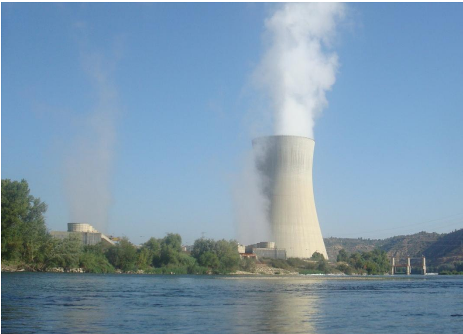
Fig. 6 Ascó nuclear power station.
