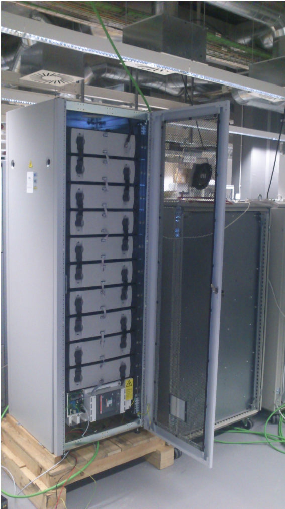
Figure D.2.: Picture of a Li-ion battery used throughout the thesis related works.
