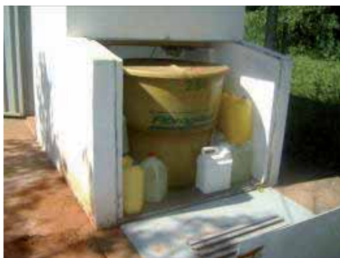
Figure 35. Chlorination tank
