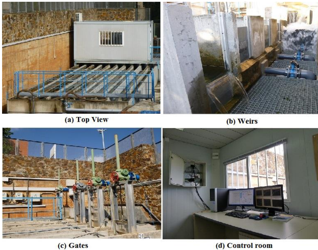
Figure 3.2 Experimental canal facility
