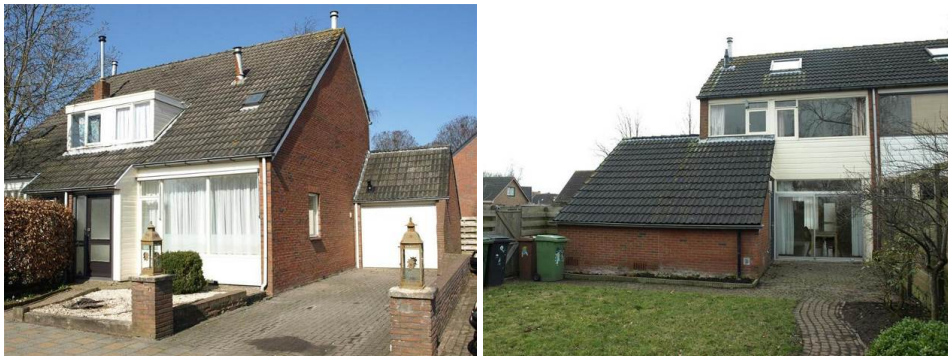
Figure 4.19: At the left side is shown a front view of the house (S-SW). Ground floor: livingroom window (room 3 ), first floor: bedroom window (room 9 ) and bath room small roof window (room 10 ). At the right side is shown a back view of the house (N-NE). Ground floor: garage and scullery (brick wall), livingrooms sliding doors, first floor: bedrooms (room 7 and room 8 ), attic: roof window (room 12 ).
