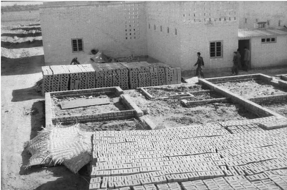
Housing Construction in Iraq (Basic Foundation Program, Iraq). Figure 3.9
