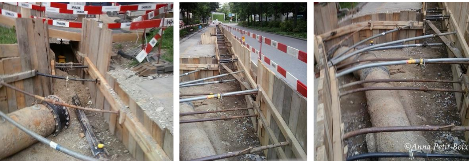
Picture: Construction of a sewer stretch in Basel (Switzerland)
