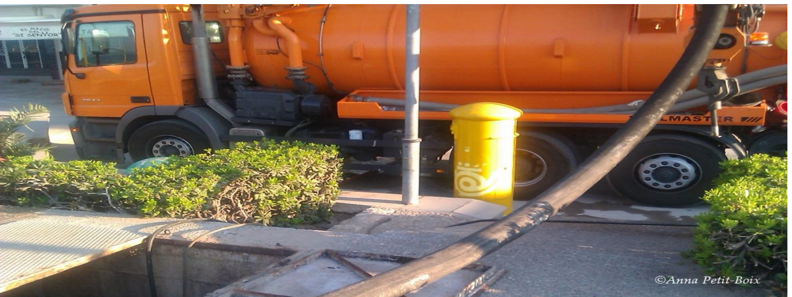
Picture: Maintenance truck cleaning a retention tank in Calafell (Catalonia, Spain)
