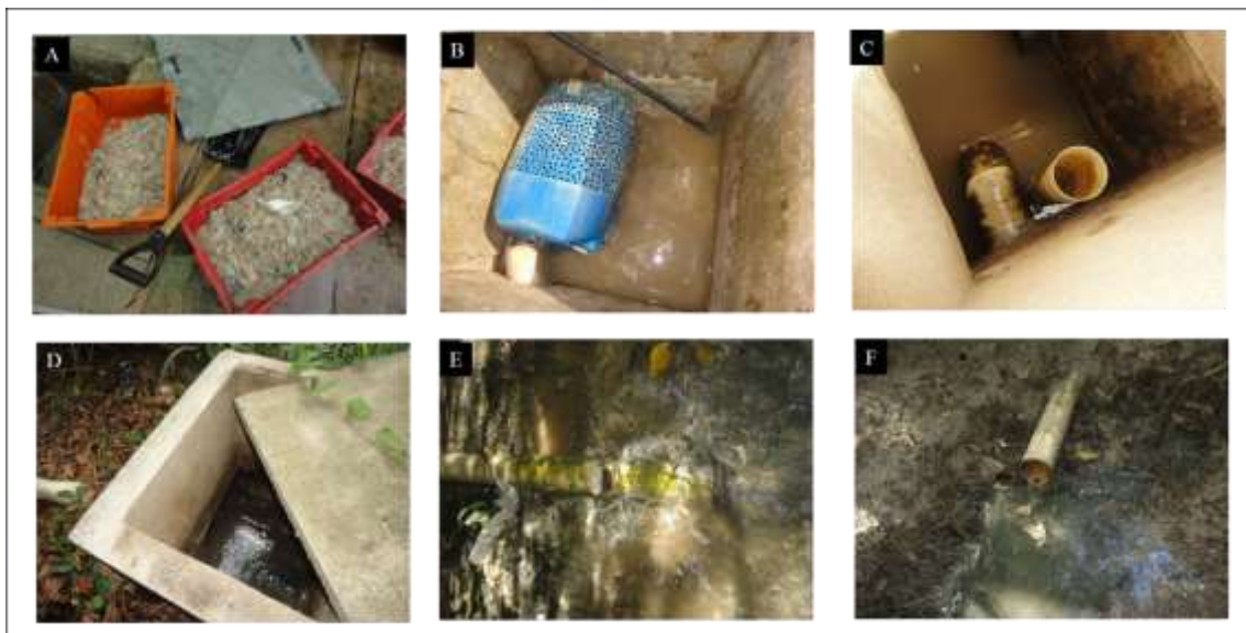
Figure 5.7: Different stages in the treatment of the residual water produced by GPesca Ltda. Removal of the solid residues (A), filtering of the solid residues (B), tank for the metabolisation of the organic matter (C), the pipeline that discharges the residual water into the Caeté estuary (D and E), effluent piped through the mangrove to a tidal creek in the Caeté estuary (F).
