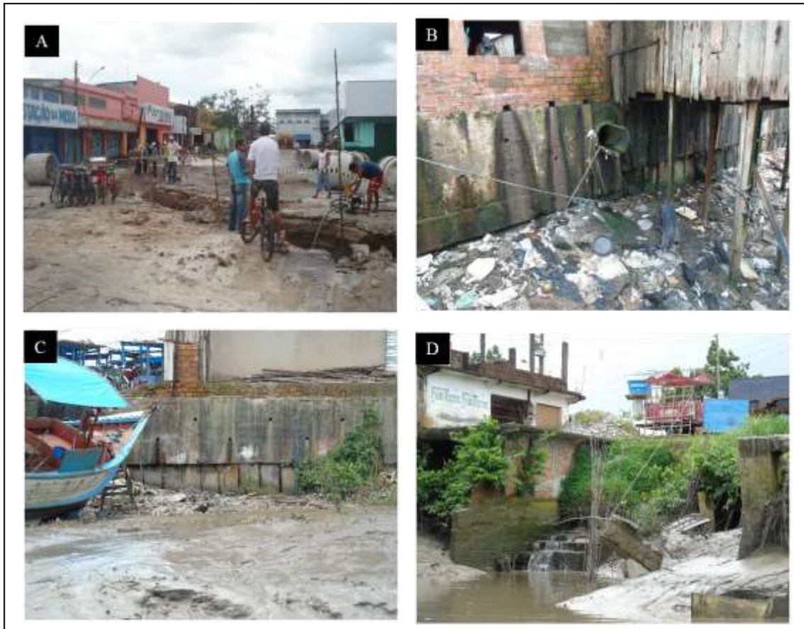
Figure 5.4: Effluent input into the Caeté estuary: sewer being channelled into the estuary (A), sewage outlets seen during low tide (B and C), and effluents channelled through open-air drains that flow into the estuary (D).
