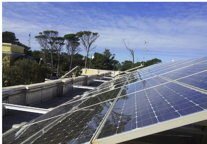
Figure 3.2. 2 Picture of the PV system showing nearby objects responsible of shadows on the array.
