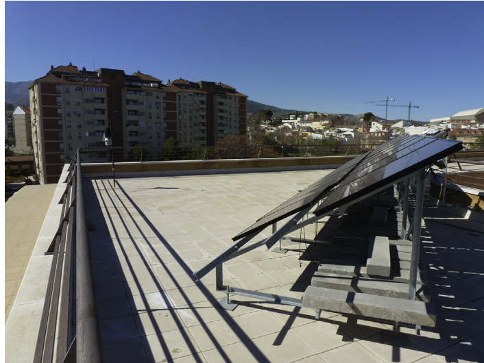
Figure 3.2. 11 PVGCS analysed in the site of Jaén. The upper row of modules comprise the a-Si:H PV field under scrutiny in this work. The lower row of modules corresponds to a micromorph (heterojunction a-Si:H/ \mu c-Si) PV field of another PVGCS.
