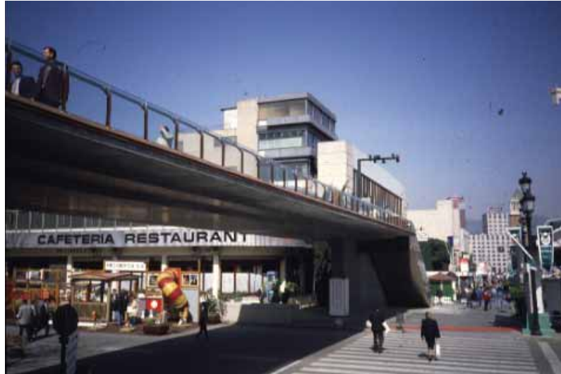
Figure 2.4: Montjuïc pedestrian bridge, Barcelona.
