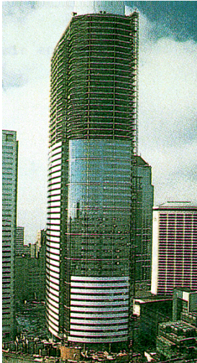
Fig. 2.3: Two Union Square Centre, Seattle
