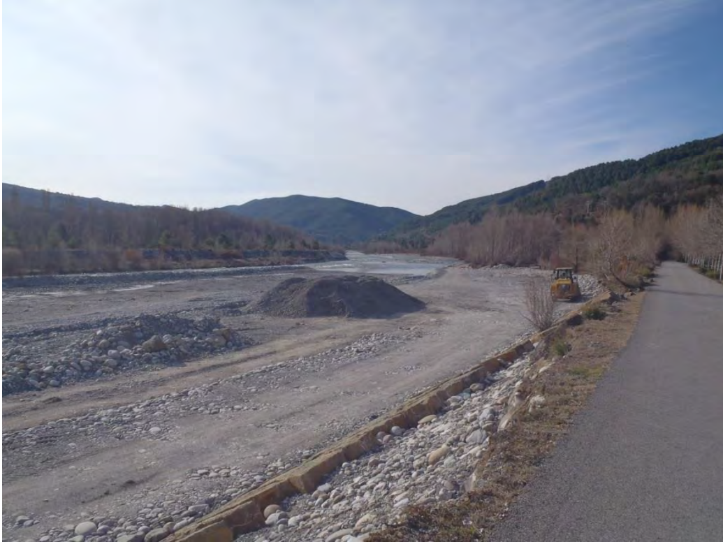
Figure 7. In-channel gravel mining for flood and lateral erosion prevention at Escalona Village in March 2013 (Damià Vericat).
