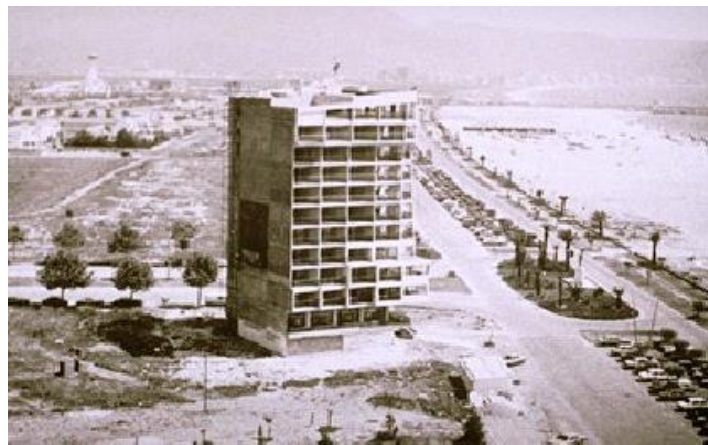
Figure 3.5 – The Construction of Delta Muga in 1983
