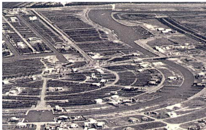
Figure 3.4 – The First Phase of Construction of the Marina in 1967
