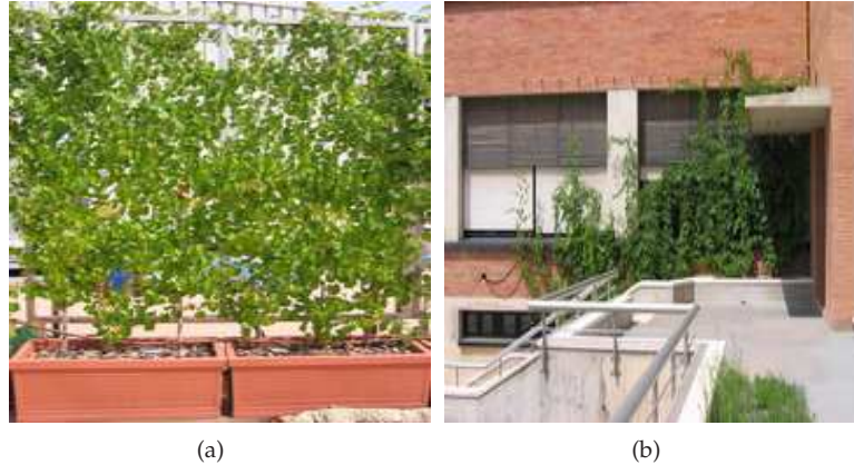
Figure 1.8: Examples of the implementation of a green curtain in a single skin facade. Deciduous vegetation allows to improve solar control during summer months, with scarce influence during winter period. The vegetation curtain also presents an additional design factor as the use of the variable leaves colours in different stages of the year.
