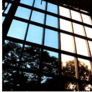
Figure 1.1: Stadparkasse building. savings bank located in Dresden, Germany. The colour of individual windows can be controlled, or the total glazing in a building can be simultaneously altered by connecting it to the building's electrical management system. This system can save up to half the energy required for air conditioning in a building. ( www.glass-resource.com/sneakpeek/sample4.htm )
