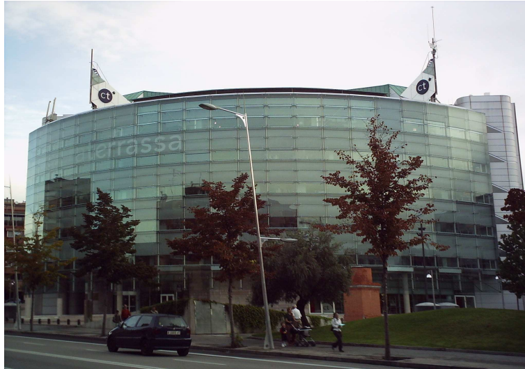
Figure 5.2: Outdoor aspect of the building
