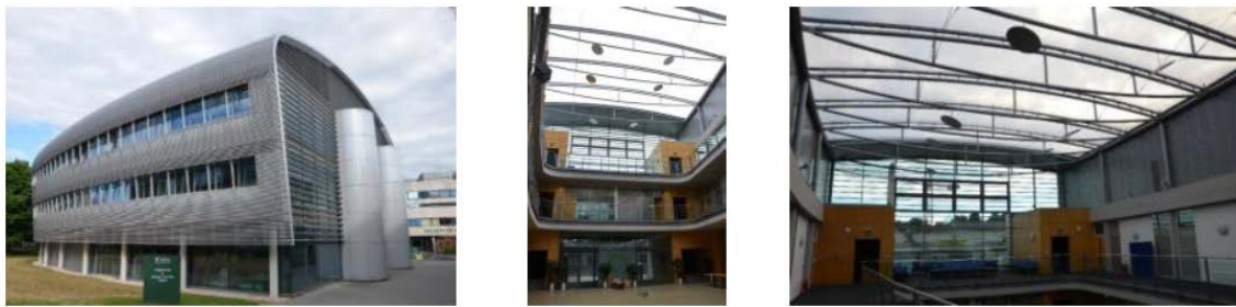
Figure 2. The external and internal views of the Engineering and Science Learning Centre at the University of Nottingham (Source: Masih et al. [66]).
