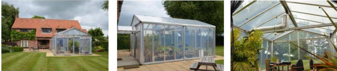
Figure 4. The external and internal views of a structure with ETFE encapsulated panels: external skin built at the garden of a detached house used as an outdoor room and a greenhouse for plants (Source: Masih et al. [66]).
