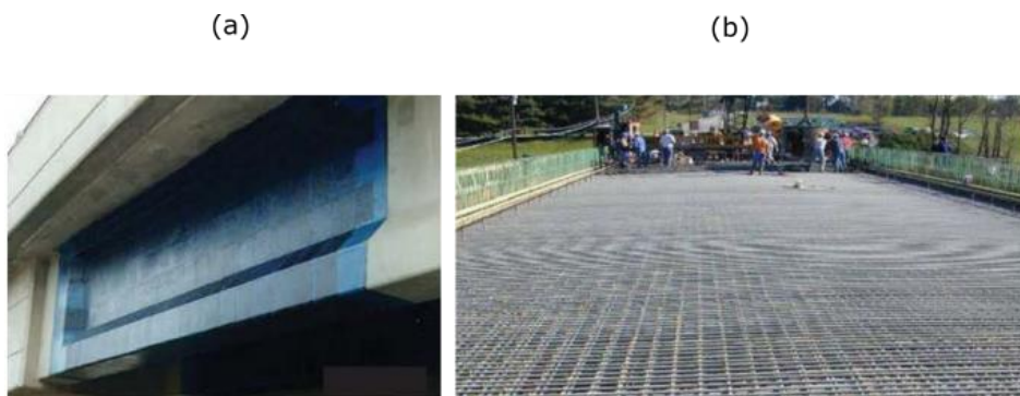
Figure 2.2: Examples of the use of FRP materials as (a) strengthening method and (b) reinforcing method [5].
