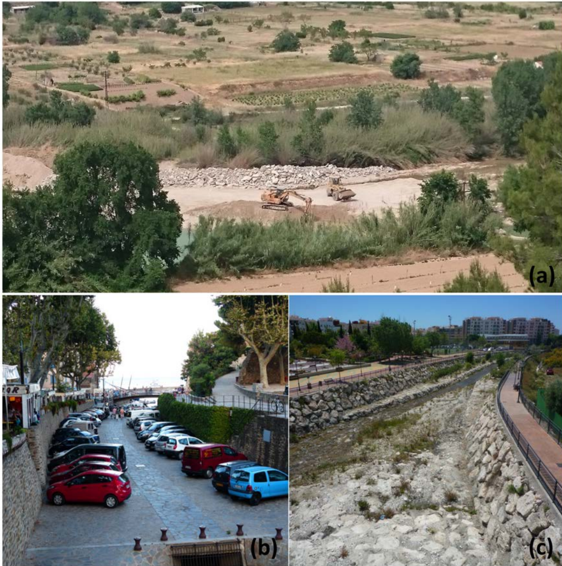
Figure 3. Examples of a TR suffering geomorphological alterations due to (a) extractions of aggregates and sediments and agriculture or (b,c) canalizations and water extractions. Photos: N. Cid and N.Bonada.
