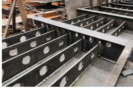
(c) Shear connector of concrete bottom slab
