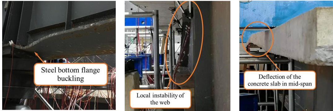
Fig. 12 Failure modes of GSP-1
