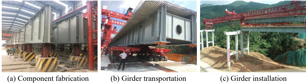
Figure 3. Pictures during the construction process
