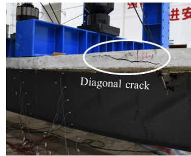
(b) Concrete diagonal crack in short span
