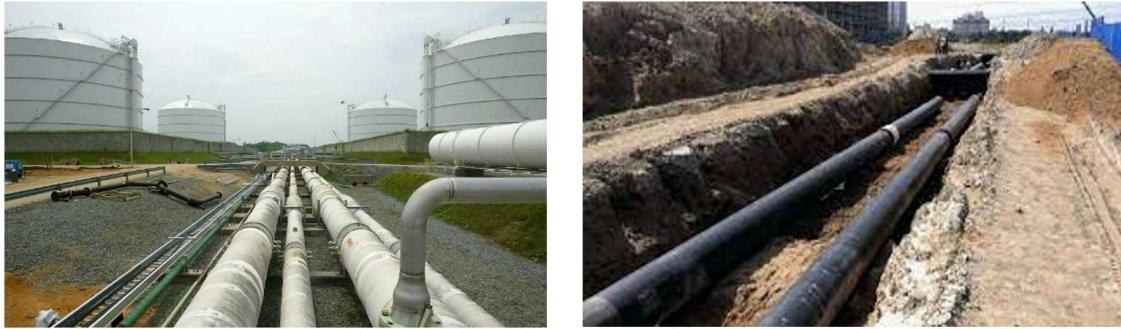
Figure 1-8. More than one pipeline in the same corridor ( https://www.passuite.com/kbase/doc/start/WebHelp_en/pipesoil.htm ).
