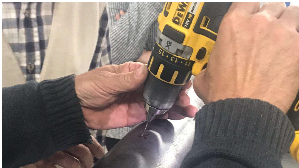
Figure 3-12. Preparing the position of a thermocouple inside the pipe wall.
