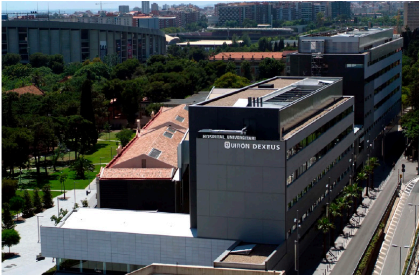
Figure 46. Hospital Universitari Dexeus; Quironsalud Group Barcelona, Spain.
