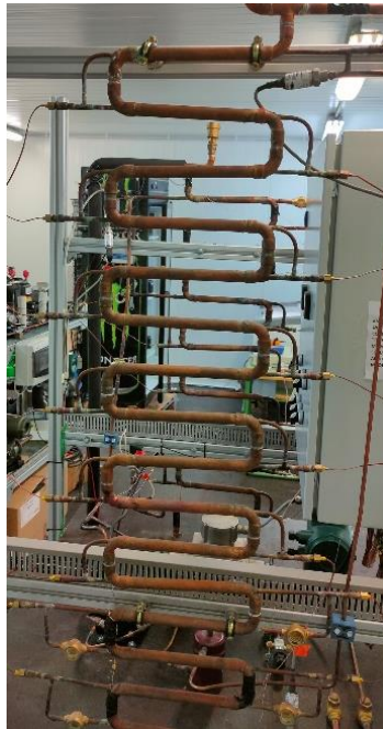
Figure 2.17. Side view of a heat exchanger showing the immersion thermocouples along its entire length.
