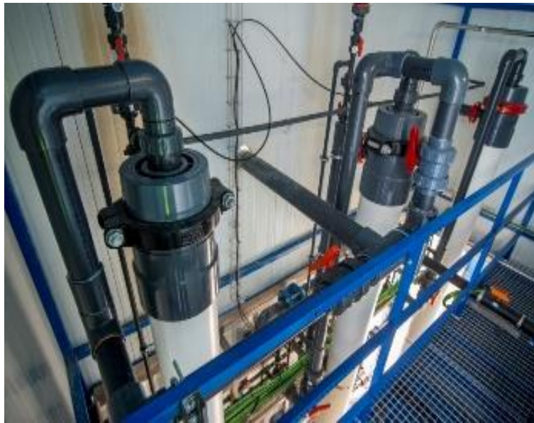
Figure 13. Description of the two external side stream tubular (PVDF) UF membrane modules (X.Flow, The Netherlands) used in the MBR prototype, which account with a total membrane area of 66 m 2 .
