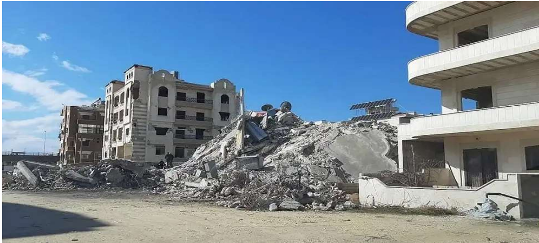
Figure 70 Lattakia city, Jableh, Earthquake, (Emarat News, 2023)
