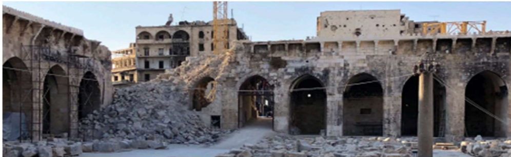
Figure 7: Great Umayyad Mosque Damage in Aleppo (Source, Bandarin, 2022)
