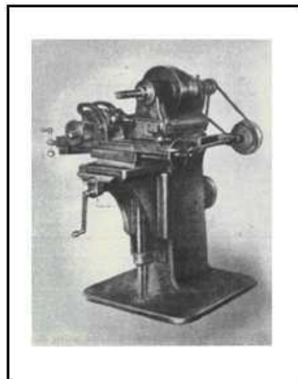
Figure 1: First milling machine built by Joseph R. Brown in 1862. Source: (Aldabaldetrecu, 2006)
