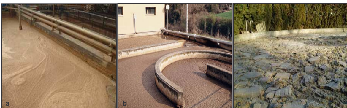
Figure 1.10 Example of foams in activated sludge systems. (a) Foam caused by nocardioforms on the aeration tank, (b) foam caused by M. parvicella on the aeration tank and (c) on clarifiers
