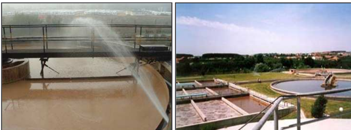
Figure 3.7 (a) non-specific control method for foam removal: use of draught water to break the scum on the surface of clarifiers and (b) specific control method: use of anoxic selector for the control of filamentous bacteria at Lleida WWTP
