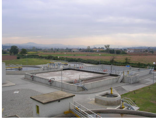
Figure 5.2. La Garriga WWTP.
