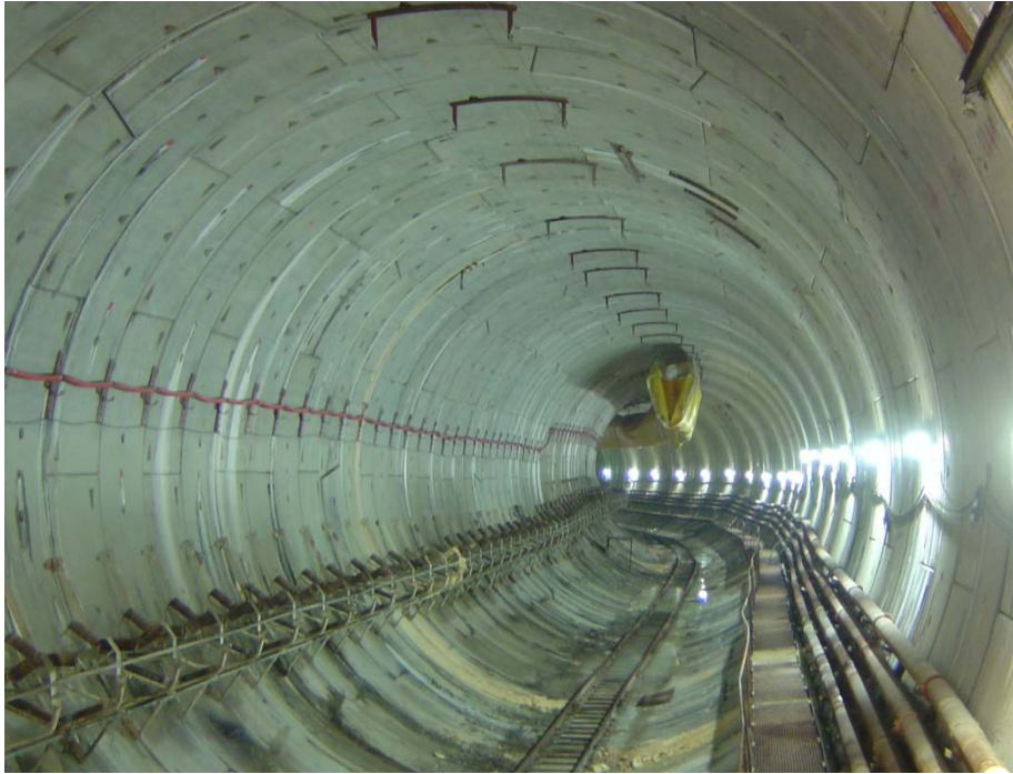
Figure 1.1. Segmental tunnel lining of Line 9 subway of Barcelona.
