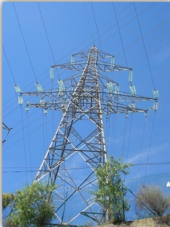
Figure 43 110 kV 4 circuits line
