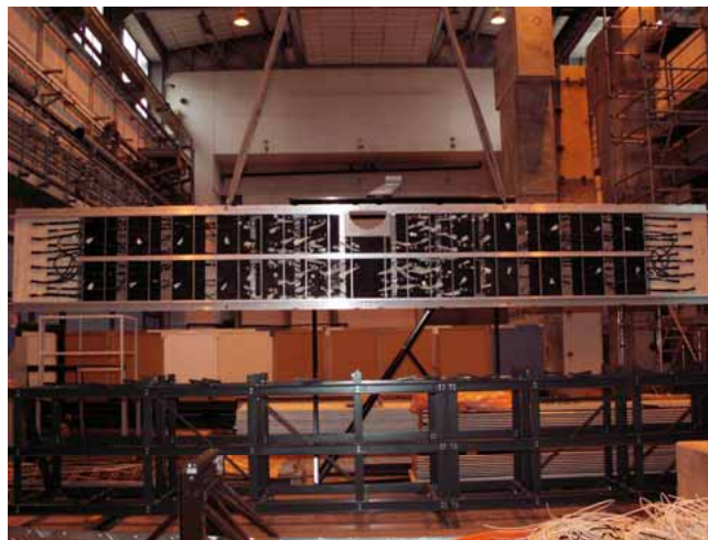
Figure 10. Supermodules under construction
