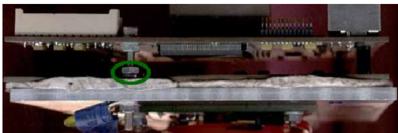
Figure 114. Nut added to improve ground connection
